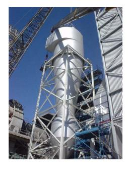
High efficiency cyclones – ferrochrome smelter
